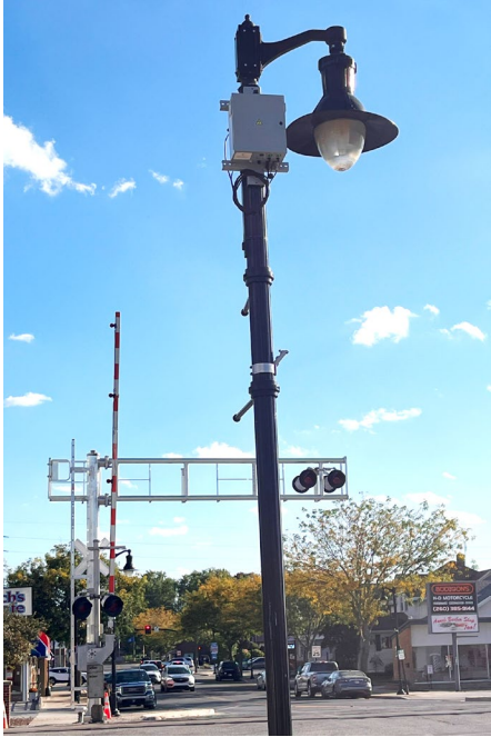
Train sensors are installed on light standards and other poles next to rail crossings and off rail property.
