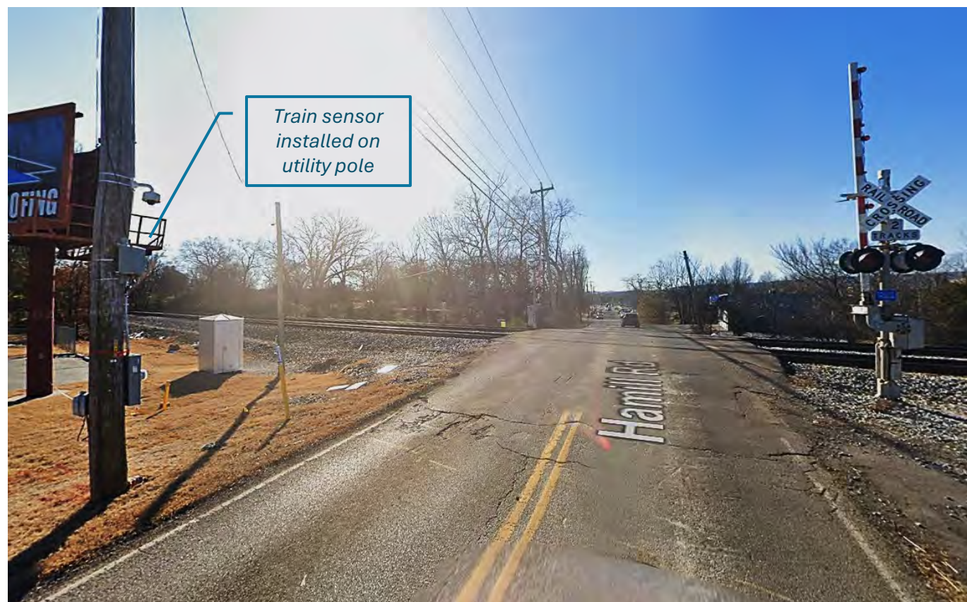
Train sensor installed on utility pole next to Hamill Rd rail crossing
