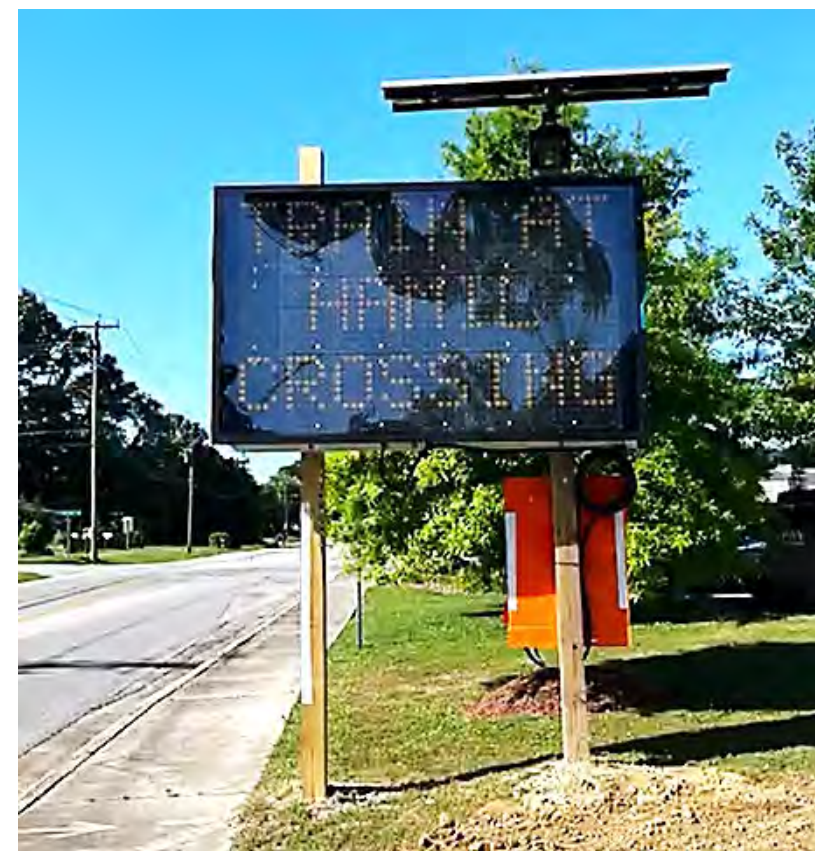
DMS board installed on Hamill Rd
