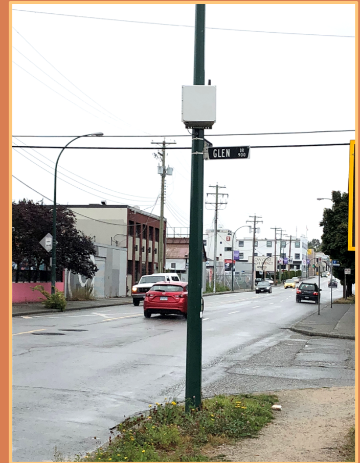
Train detection sensor installed on light standard next to rail crossing
